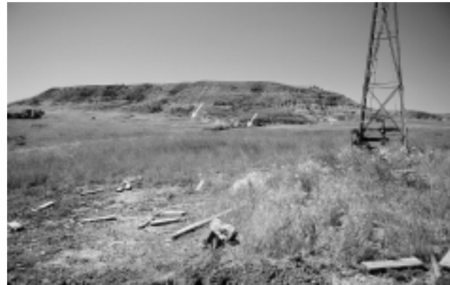
Photo taken looking south-southwest to Coal Butte in Emmons County. The mine entrances were located on the northeast corner of the butte (arrows). The mined seam outcrops along the hillside about 20 feet below the windmill in this photo.
