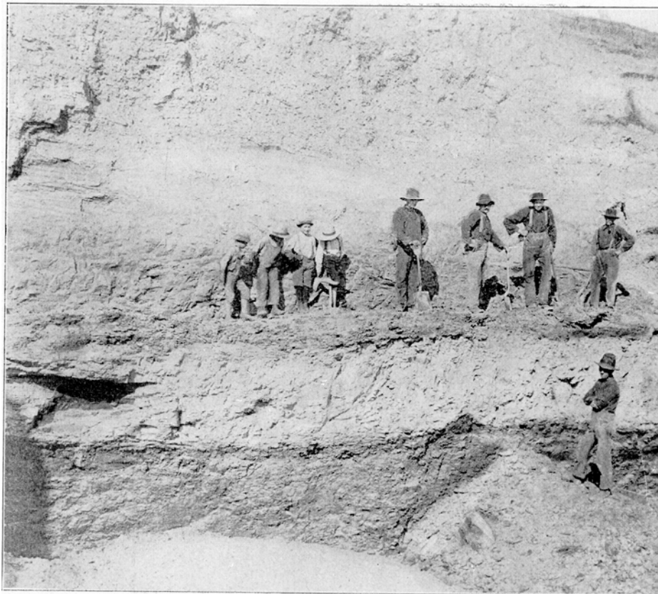
Lignite in the Pit of the Dickinson Fire Brick Company. The Upper Clay Is Used for Brick While the Lignite is Used for Fuel in the Kilns.
